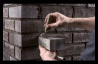
The vertical joints can be finished more easily with a smaller pointing trowel.
